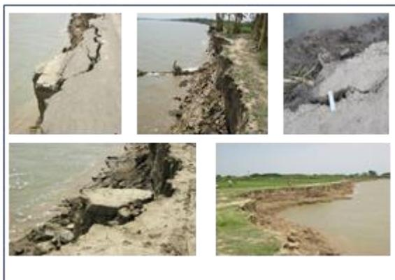
**Fig 2:** Some photographs of bank failure in Sundalpurchar and Gosainchar
